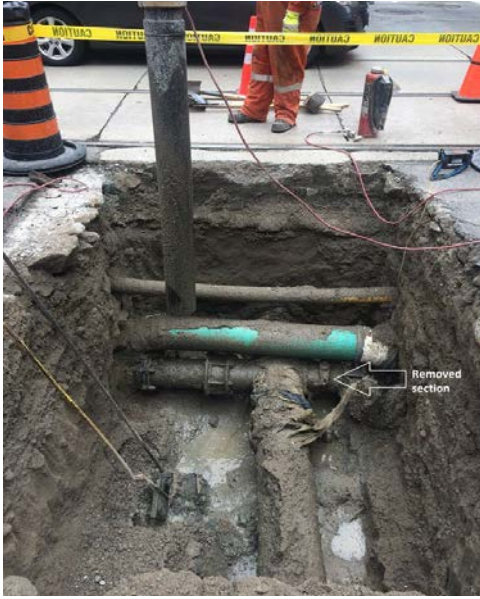
Figure 5.2-14: Leak Investigation on Vintage NPS 12 Gas Main
