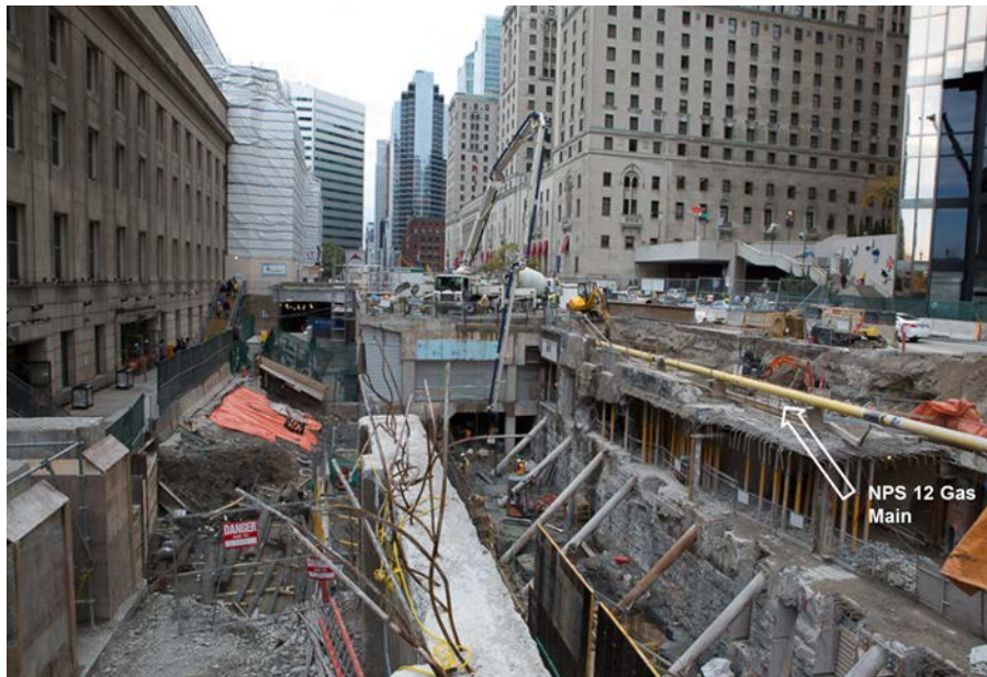
Figure 5.2-10: Long Section of NPS 12 Gas Main Exposed at Major Construction Site in Toronto
