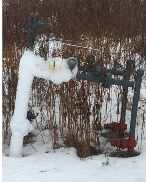
Figure 5.3-10: The Joule-Thomson Effect on a District Station
