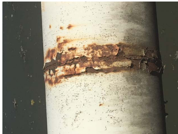
Figure 5.2-23: NPS 20 Pipe Crossing Exhibiting Corrosion
