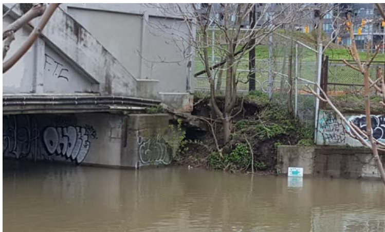
Figure 5.2-19: NPS 30 Pipe Bridge Westerly Abutment Undermining
