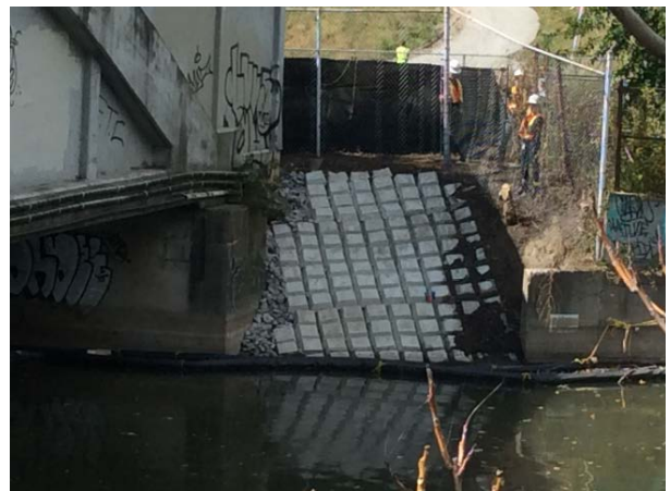
Figure 5.2-20: Temporary Remediation to the Undermined Abutment
