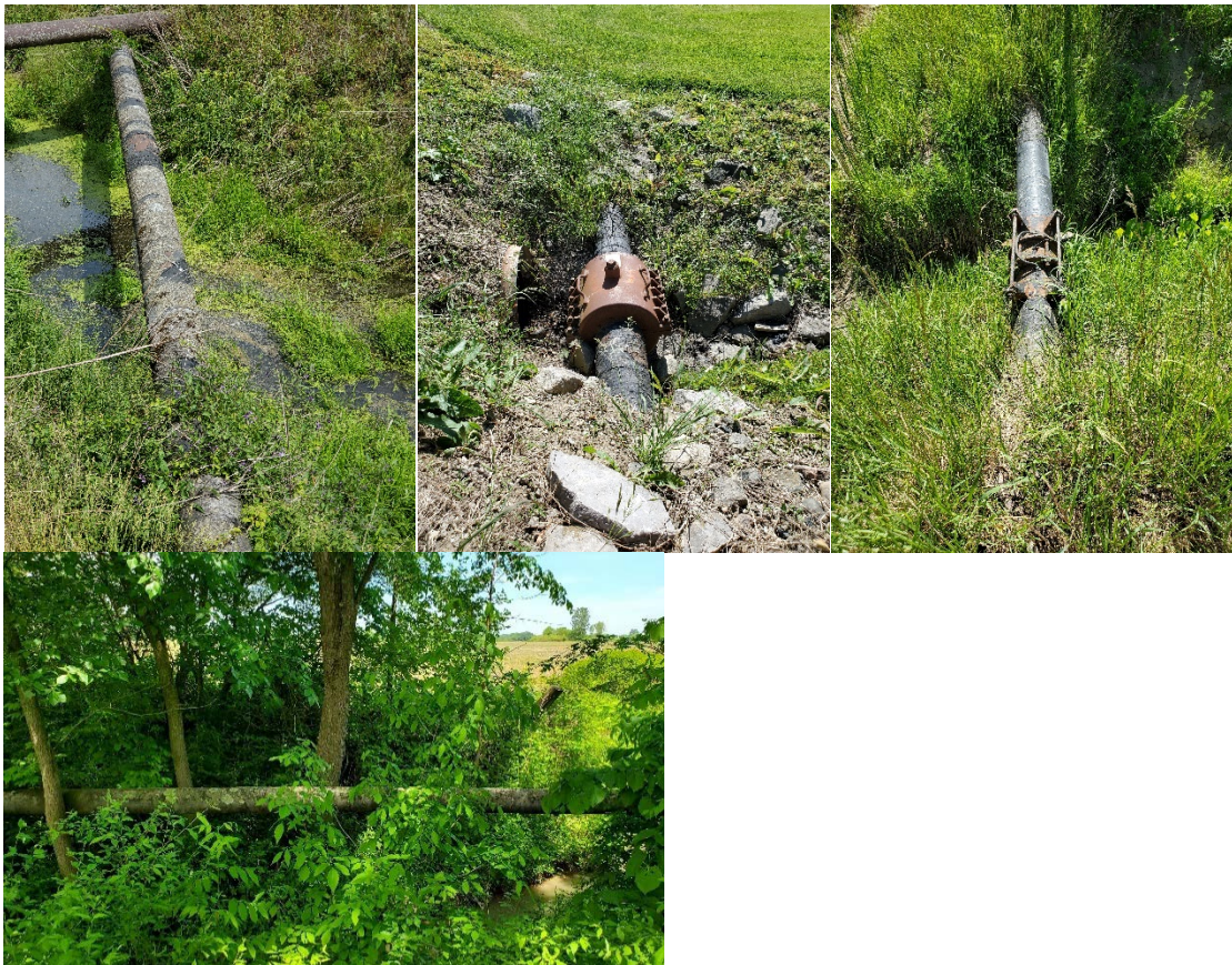
Figure 4-1 Examples of London Lines Exposed Piping (June 2020)
