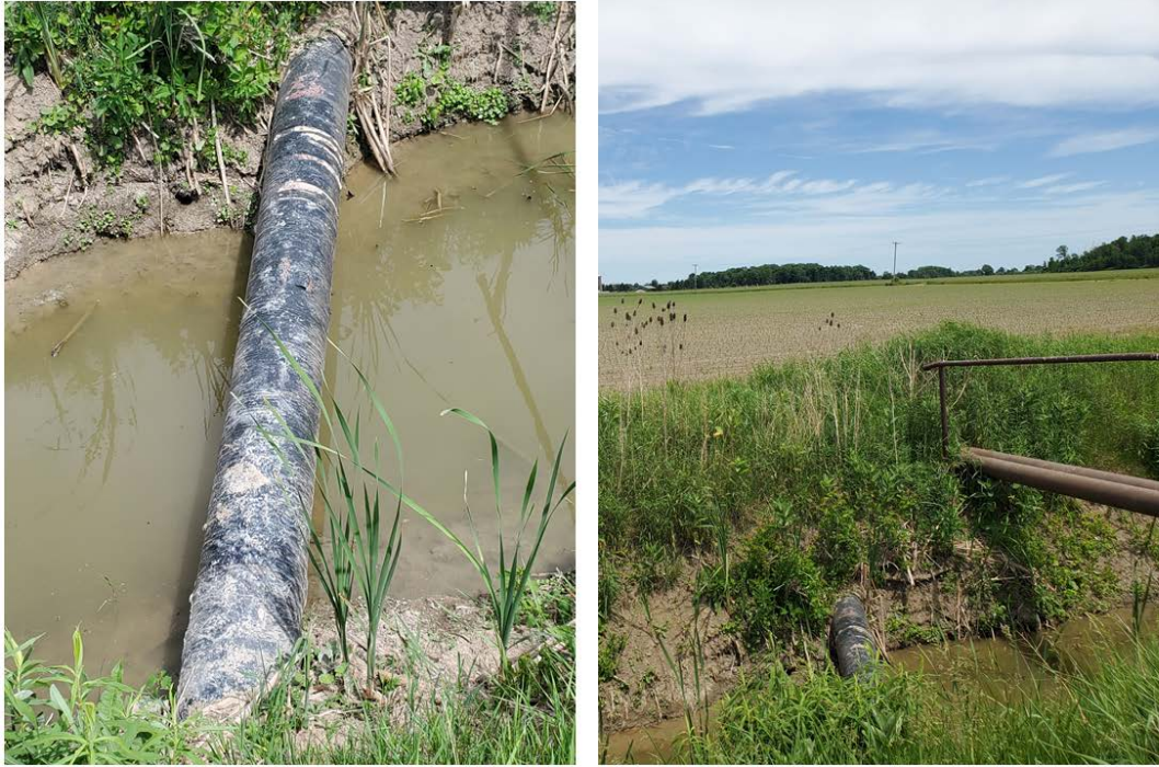
Figure 6: Aerial Crossing and bridge used for inspection, prone to partial submersion (Pratt Siding and Knapdale, through private easement). Left is a close-up, right show the crossing in context.
