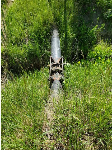
Figure 3: Aerial Crossing, with “restrained” Dresser Coupling (Bentpath Line, between Tramway Rd and Esterville Rd) indicating severe deflection and mis-alignment of the pipe. Left is a close-up, right show the crossing in context.
