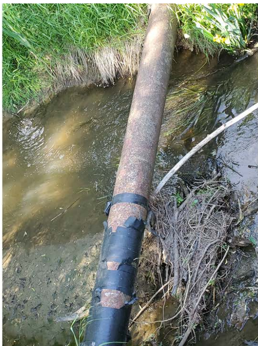
Figure 9: Aerial Crossing with peeling pipe coating (Falconbridge Dr, east of Christina Rd). Left is a close-up, right show the crossing in context.
